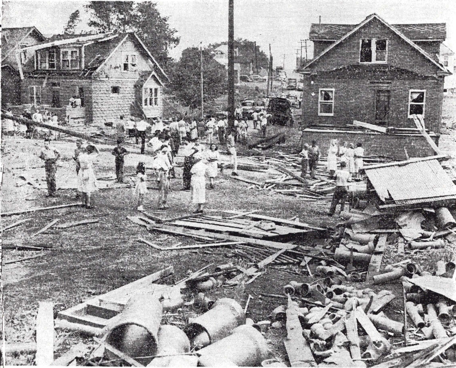
above is a general view of Pittsburgh street and Shady avenue. Burgettstown, which was hit with demolishing force. Materials from the Pappas lumber yard are shown strewn about the area. Lumber and debris, including 2x4s were picked up by the sweeping
